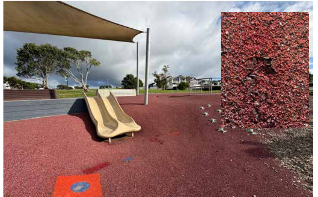
The rubber chip surface at Constellation Park in Beachlands has started to degrade, prompting environmental concern.
